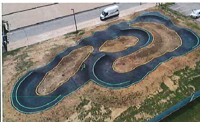
Pumptrack de 1000m 2 - France
