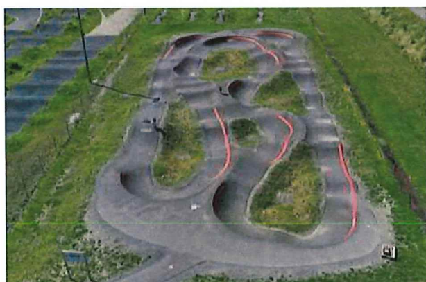
Pumptrack de 1200m 2 – Aigle
